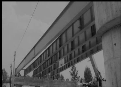
TLAPACOYA BRIDGE MX-PUEBLA HIGHWAY
